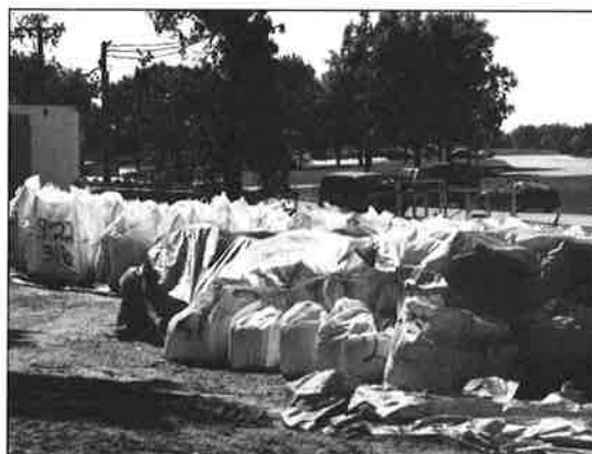
These reinforced polyethylene super sacks, filled with contaminated soil, are ready to be shipped.
